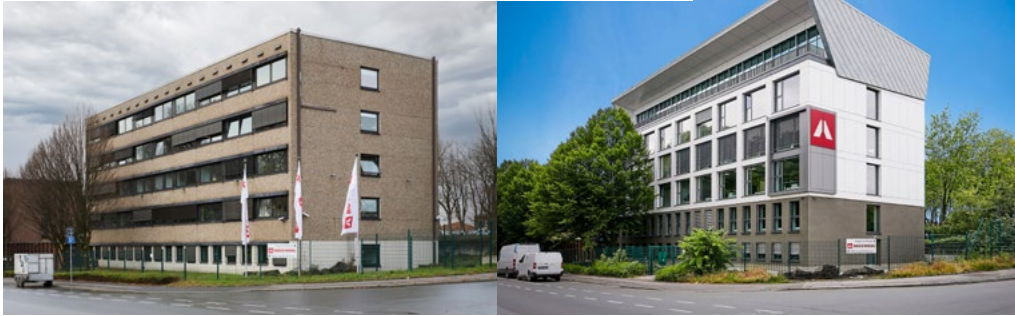
ROCKWOOL's administrative office in Gladbeck, Germany before and after renovation
